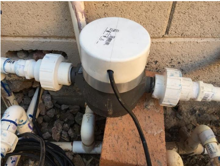
The resulting assembly came out nice but in the future I hope to be able to simplify the interface hardware and go with a proximity switch that can sense the spinning steel bar. The proximity switch I tried did not work.
