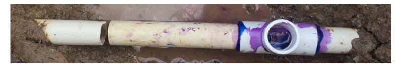
Instead, I cut the pipe on the right and cemented in my T. Then I cut the pipe to the left and shortened it so when cemented into the left side of the T, there was a ¼" gap.
