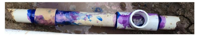
The final step was to apply primer and cement to the pipe ends plus to the sliding coupler. Deflect the pipe, slide on the coupler on the right pipe end, release the deflection, and slide it to the left until it is centered over the gap. With fresh cement, the coupler slides smoothly and with little resistance.
