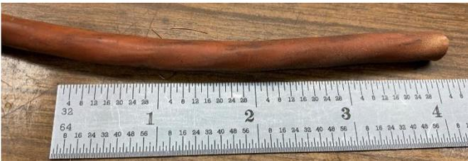
The first step is to remove 4-inches of sheath from one of the cables.
