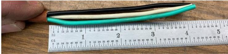
Pulling off the sheath pulls some of the wire out of the cable so I had to trim the exposed wires back to 4-inches.
