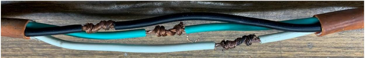
There are a few critical things missing in this picture<sup>3</sup>. I have not soldered nor insulated the Western Union splices. The shrink tubing around the entire joint was not installed. Please do all three of these if you plan to follow my procedure.
