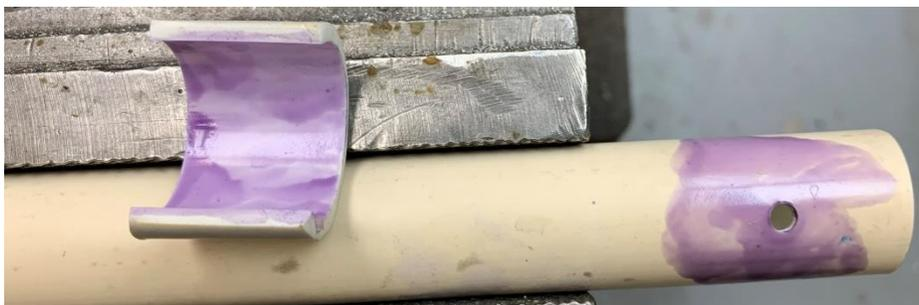
To use the patch, I first apply primer to the inside of the patch and the outside of the pipe being patched.
