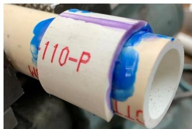
The setup time is a function of the type of cement used and the ambient temperature. I prefer to give the joint around 2 hours before applying pressure. Since the patch self clamps, at least I'm not tying up any tools while I wait.
