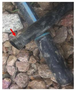
I bumped a nearby coupler and the soft pipe fell off. Note the compression in the pipe. It is very close to the end. The installer were supposed to push the soft pipe into the coupler about one inch. Well, I need to get it back in.
