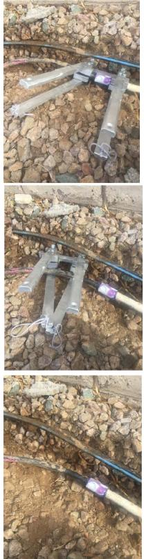
Here you see the tool has been placed in a trench. The hard pipe with coupler and collar rests in the right set of jaws. The soft pipe rests in the left set of jaws.
