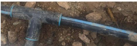
Success! The soft pipe is now in about an inch. I then pushed the soft pipe connected to the left arm of this T in about another half inch. One obvious improvement to this tool is to have the pipes load from the other side of the pivot. Then the user could place this tool around the pipes similar to using a pliers.
