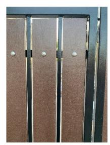
Using my table saw, I ripped 18 planks<sup>4</sup> 3½ inches wide and the remaining four 3 inches wide. All were cut to a length ½ inch less than the inside distance between horizontal bars. This gave me a 1/8-inch gap around each slat.
