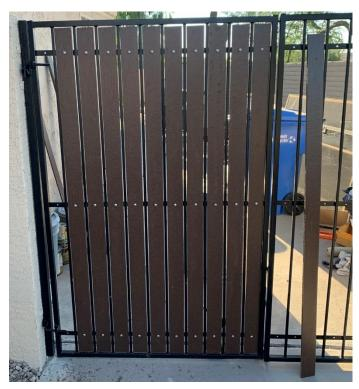
Using 1-inch ¼-20 carriage bolts, I loosely secured the tops of all slats on one gate. This weighed down the frame and made it relatively square.
