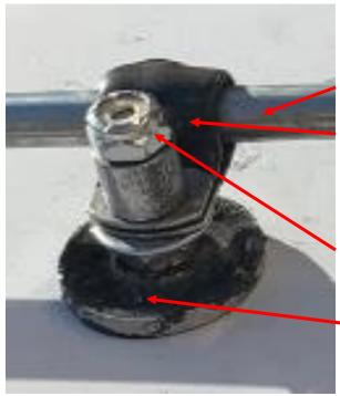
A 1/4-inch diameter steel rod is clamped to the screw.
