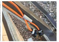
Squeeze the first cable through the left end of the retainer. Then bend it slightly to get through the right end of the retainer. Repeat with the second cable. Cables retained!
