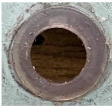
How about making cast-in-place grommets? They are always a perfect fit for the hole regardless of plate thickness. Yes, it looks a bit rough, but it certainly protects wires that pass through it from the edges of the plate.
