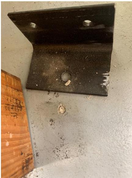
I drilled down just enough to form a shallow hole in the concrete. Then I was able to finish drilling with the bracket out of the way.
