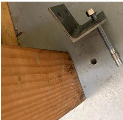
After vacuuming out the hole and the floor around the leg, I fitted the bracket with the concrete anchor.
