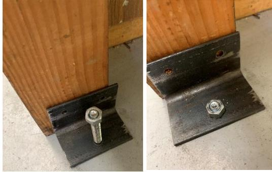
Using a large hammer, I drove the concrete anchor down until the nut contacted the top of the bracket. Then the nut is tightened to lock in the anchor.
