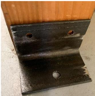
After verifying that my workbench was exactly where I wanted it to stay, I placed my new bracket against its 4 by 4 leg. That  $\frac{3}{8}$  inch hole tells me exactly where to drill the concrete.
