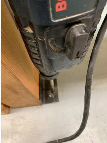
Using my Bosch hammer drill, I begin drilling the concrete through the bracket hole.
