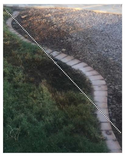
Then I turned the drill around and went under the bricks. About every 4 feet I dug a small hole in order to verify I was going in the right direction.
