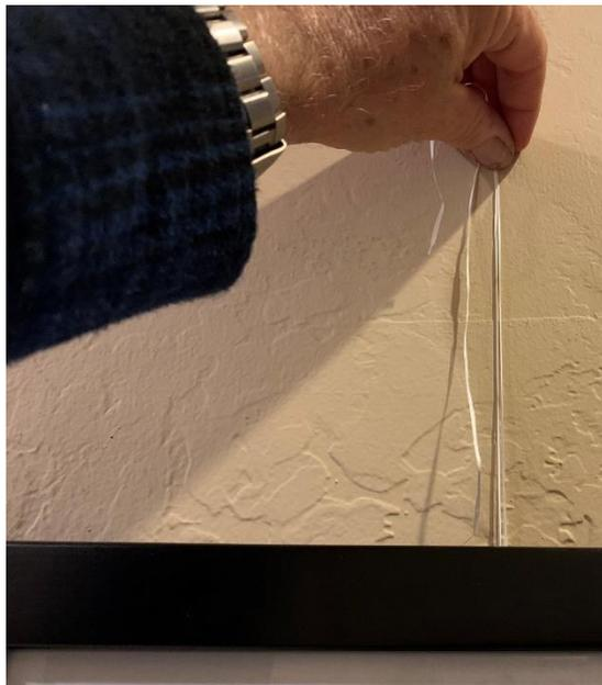
While pulling up on the floss, I lower the picture such that the the bail slides along the threads until it engages with the screw. With the picture securely supported on the screw, I pull one end of the floss straight up and out. Done.
