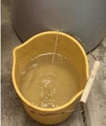
My first step was to drain as much water out of the tank as possible. At first, I used a siphon but it was too slow plus couldn't reach the water below the salt line. So instead I drilled a hole in the tank a bit higher than my shortest pail. Look closely and you will see a ¼" diameter stream shooting into the yellow pail. Periodically, I would put my finger over the hole, dump the pail into a taller bucket, and repeat. In no time, all water above the hole was out.
