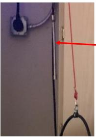
The weight is a slender steel bar that does not tangle with the power cable.
