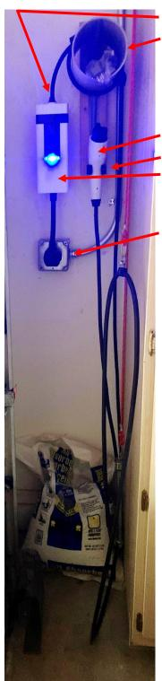
The charging cable exits the top of the Charging Station, loops around a piece of 6-inch diameter ABS pipe twice, and then drapes towards the floor. The ABS pipe ensures the cable's minimum bend radius of 3 inches is not violated.
