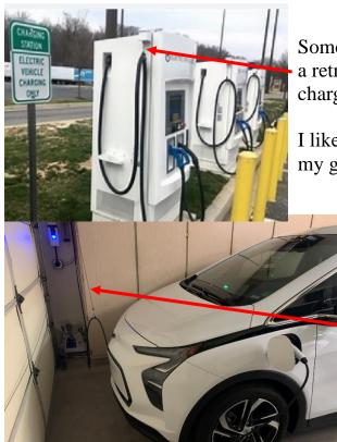
Some Electric Vehicle charging stations have a a retractable cable that helps to support the charging cable.
