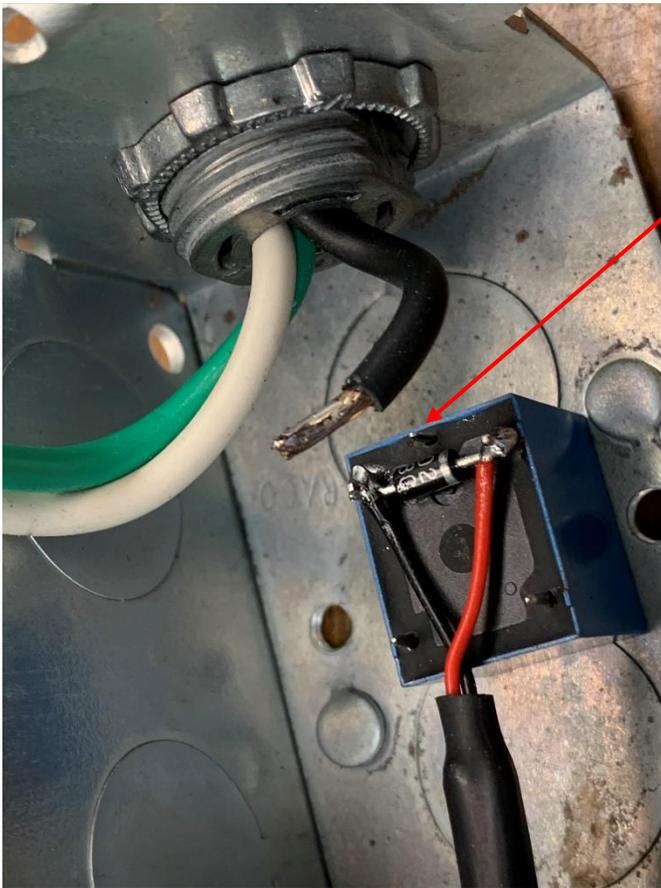
The power cord is fed through its cable clamp.
