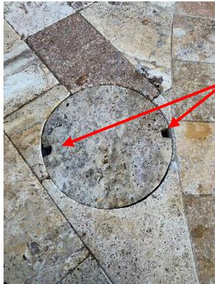
This access cover is surprisingly heavy. It is cut from rock and is about 1 inch thick. Lifting it out requires sticking a finger down each square hole. Not only is this a bit hard on the fingers, there are a number of spiders down there and some bite.
