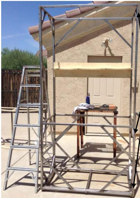
The fasteners are part of a structure that is occasionally set up in various places and then knocked down into 4 flats for transport and storage. It is 2' deep, 4' wide, and 8' tall.
