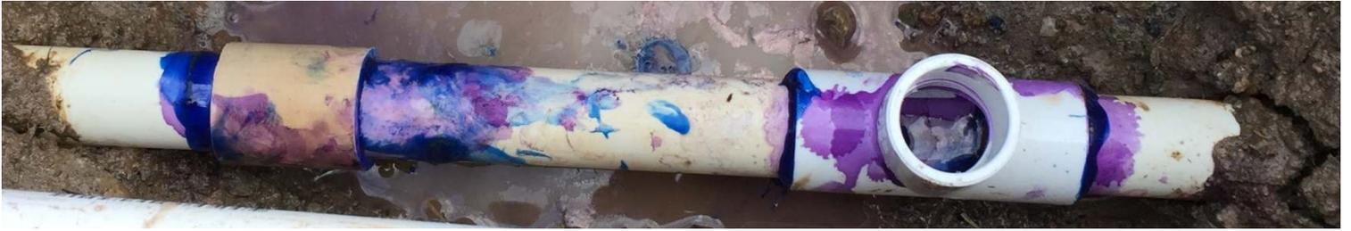
The final step was to apply primer and cement to the pipe ends plus to the sliding coupler. Deflect the pipe, slide on the coupler on the right pipe end, release the deflection, and slide it to the left until it is centered over the gap. With fresh cement, the coupler slides smoothly and with little resistance.
