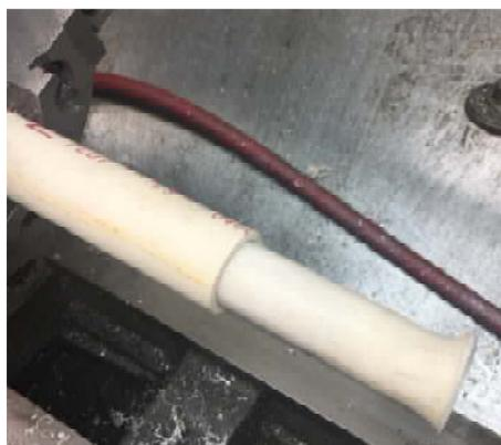
Using the pipe that will later be used in the repair, I slightly expand the ID of the heated pipe. Push the tool in at least 3 inches.
