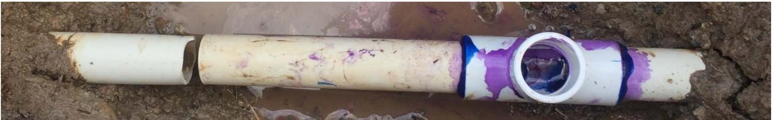
Instead, I cut the pipe on the right and cemented in my T. Then I cut the pipe to the left and shortened it so when cemented into the left side of the T, there was a ¼" gap.
