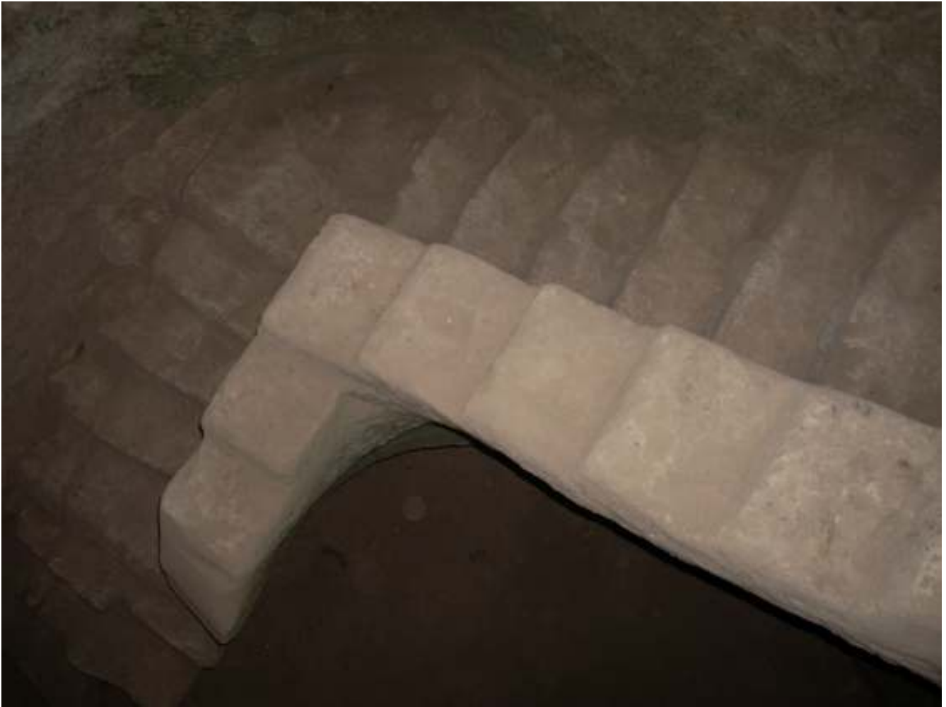
These stairs were very easy to climb. All of it was carved from the existing rock.
