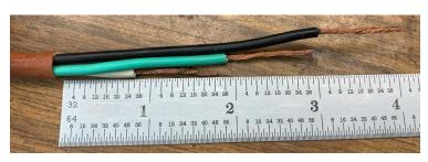
I then stripped 1-inch of insulation from the end of the black wire. The green wire was trimmed to 3-inches long and 1-inch of insulation was removed from it. And finally, the white wire was trimmed to 2-inches long and 1-inch of insulation from removed from it.
