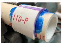
The setup time is a function of the type of cement used and the ambient temperature. I prefer to give the joint around 2 hours before applying pressure. Since the patch self clamps, at least I'm not tying up any tools while I wait.
