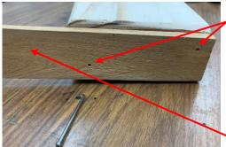
I predrilled two holes in one of the shims to prevent splitting before driving finishing nails.
