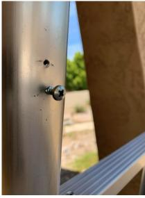
I installed a sheet metal screw in each hole.
