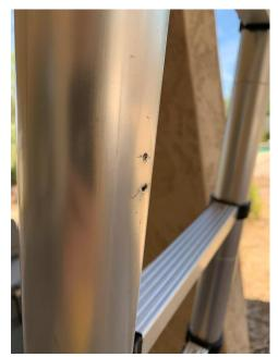
With the ladder fully extended, I drilled a 1/16<sup>th</sup> inch hole in the center of each dent. You can't see the dents here because I had low confidence that this would work, so I didn't bother to document it.
