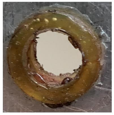
This close-up shows how the grommet fully covers the edges of the plate. The hole is <sup>1</sup>/<sub>4</sub> inch in diameter.
