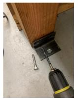
With the workbench back in the desired position and the bracket secured to the floor, I used the drill that matches the body of the screw. Remember that I last used this drill to open out the two adjacent holes.
