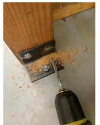
The first screw is then installed and fully tightened.
