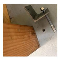
After vacuuming out the hole and the floor around the leg, I fitted the bracket with the concrete anchor.
