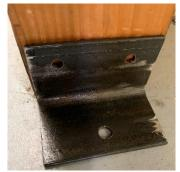
After verifying that my workbench was exactly where I wanted it to stay, I placed my new bracket against its 4 by 4 leg. That 3/8 inch hole tells me exactly where to drill the concrete.
