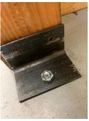
Using a large hammer, I drove the concrete anchor down until the nut contacted the top of the bracket. Then the nut is tightened to lock in the anchor.
