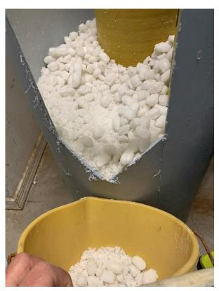
It was time to get "medieval" on this problem. I sawed a slot in the side of the bin with a V at the bottom.
